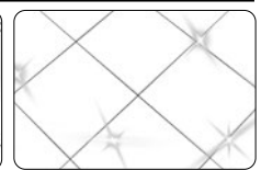
Tiles and grout are now clean.
