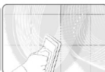
Immediately start scrubbing wall area
